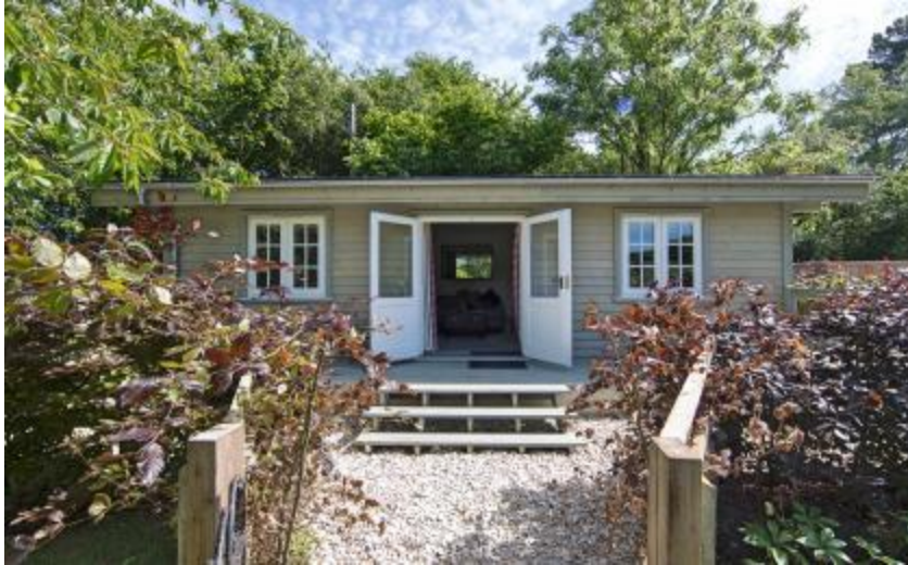
Front steps and entrance to The Hedgerow
